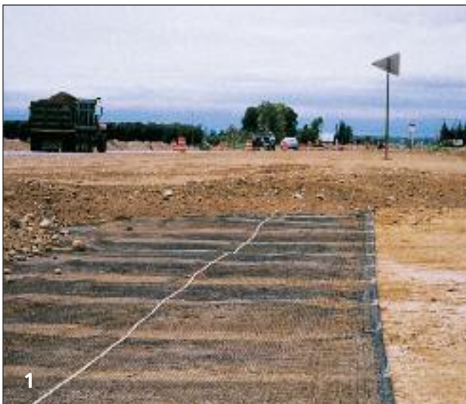
Photo 1 + 2: Base reinforcement with Fornit® geogrids.
