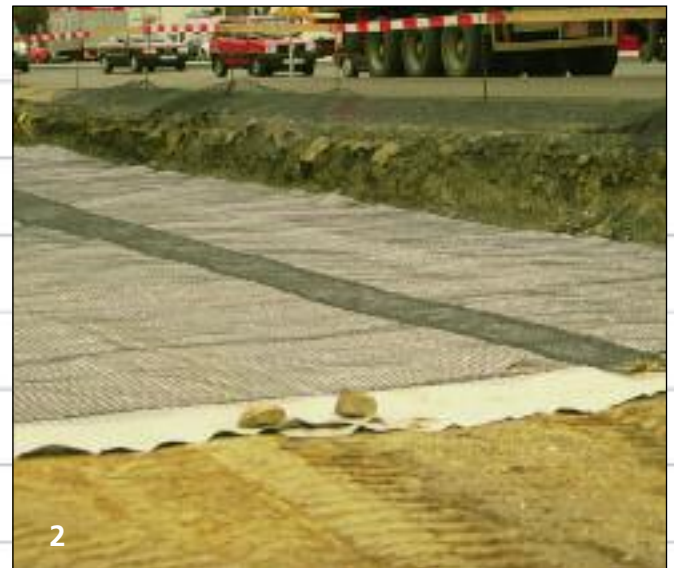
Photo 1 + 2: Base reinforcement with Fornit® geogrids.
